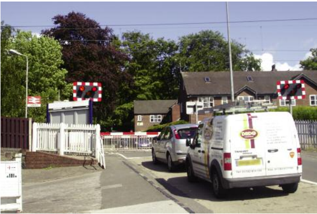
A full barrier level crossing in operation
